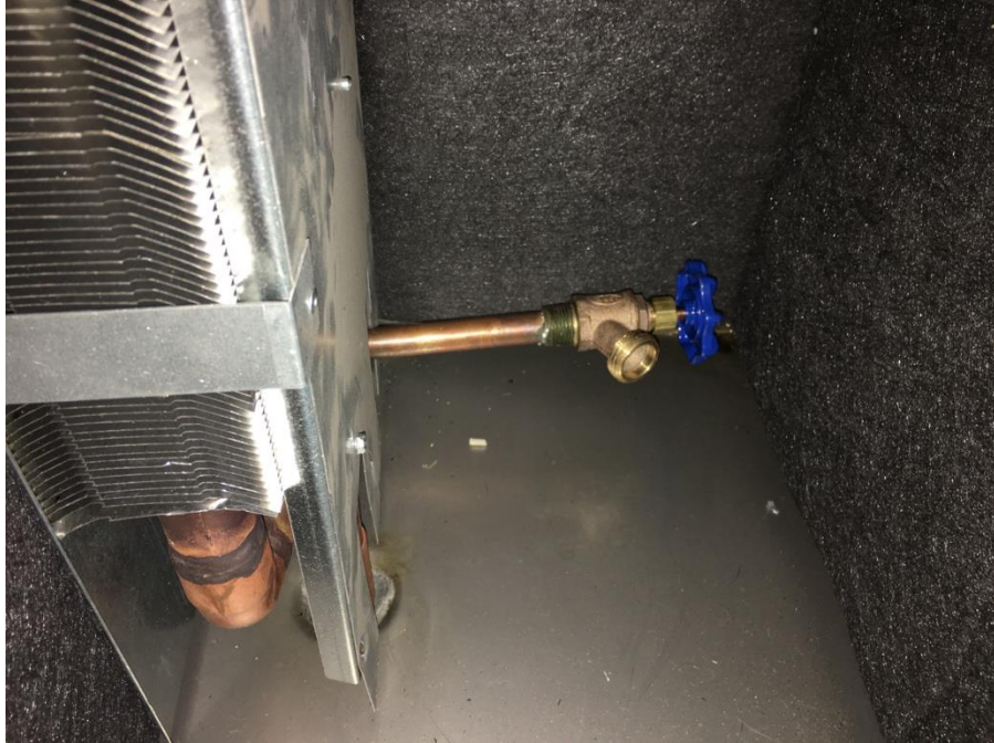
Bottom U-Bend with drain valve
