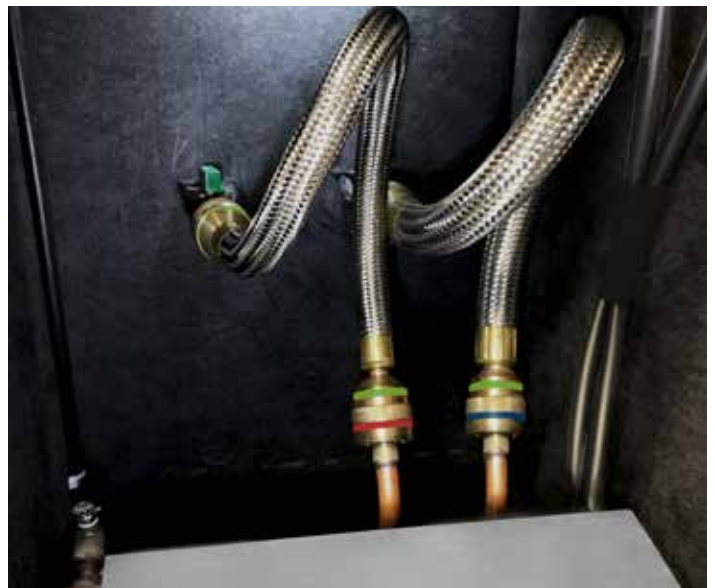
Audible lock indicator assures a connection has been made.
