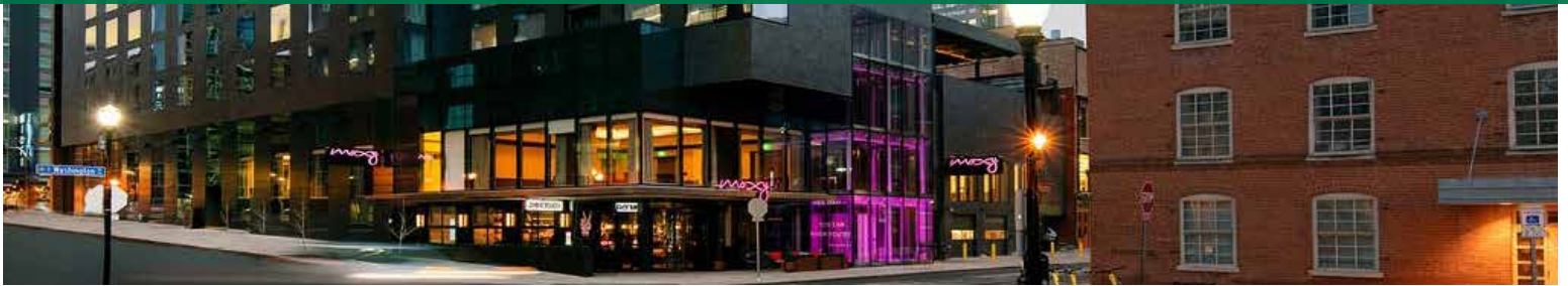
Moxy Hotel, Louisville, KY - 340 Intelli-line® Units
